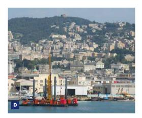
challenge was handled successfully in partnership with Terramare, the Boskalis Finnish subsidiary. The backhoe Maricavor and two Terramare blasting pontoons removed a total of 110,000 m³. The dredged material was also used for the reclamation of land for the container terminal of Calata Bettolo. This optimized the construction processes by achieving a range of construction goals at the same time.
