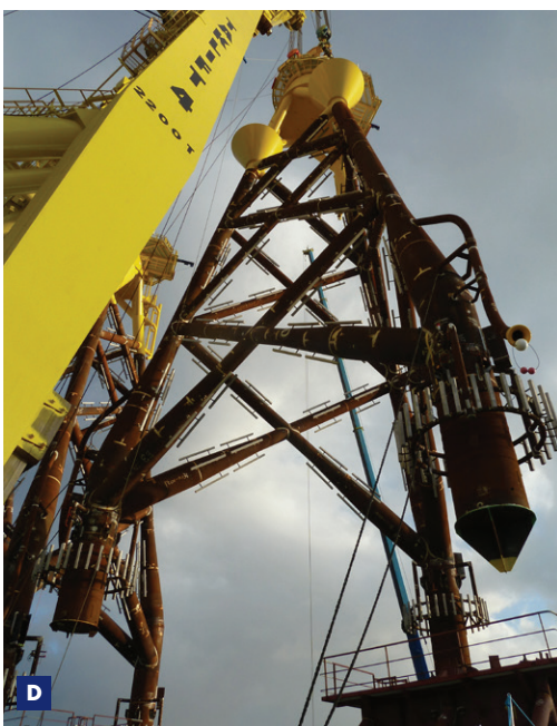
D Taklift 4 load-out jacket at Trelleborg E Taklift 4 commencing jacket installation
