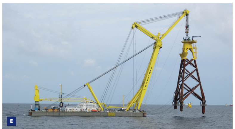
D Taklift 4 load-out jacket at Trelleborg E Taklift 4 commencing jacket installation
