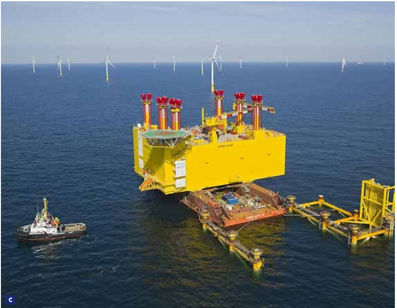
C SylWin Alpha converter station topside
