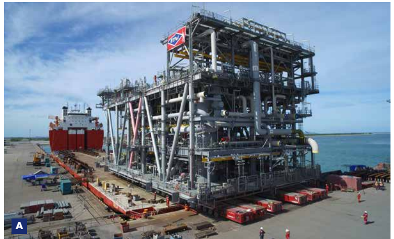
A FINESSE - Loadout of large module in Thailand
