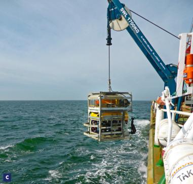
Boskalis decided to cut the piles internally to avoid the excessive amount of dredging (and consequent seabed disturbance) required for external cutting. Together with DECO Subsea Services Boskalis developed, built and tested a grout dredging tool to remove the grout from the piles. The tool used a combination of mechanical cutting wheels, high-pressure water jets and an airlift to disintegrate and remove the grout and soil plug inside the piles to the required depth.
