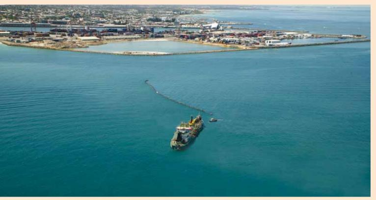
Trailing suction hopper dredger Cornelis Zanen pumping ashore the dredged material for the extension of the Rous Head Container Terminal in the port of Fremantle
