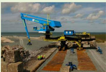
The 'blockbuster', a specially developed crane used to place the large blocks to construct the 'movable' flood barrier
