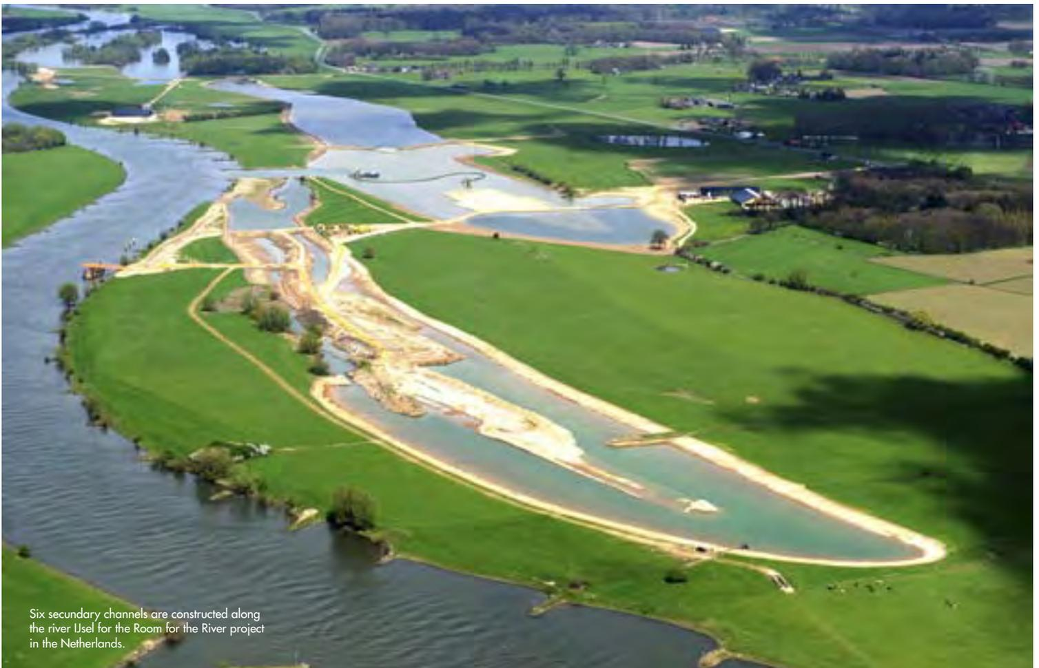
Six secondary channels are constructed along the river IJssel for the Room for the River project in the Netherlands.
