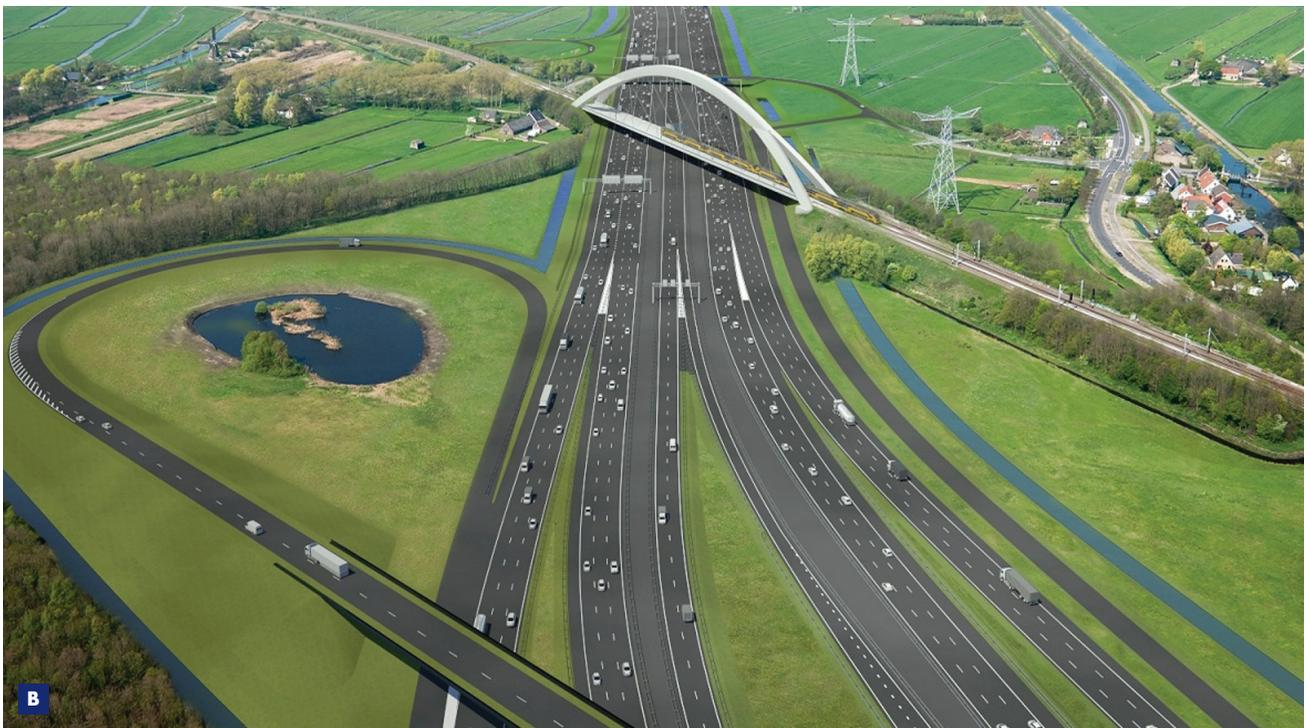
crossing the Amsterdam-Rhine Canal, the doubling of the Hollandse Brug bridge across the Gooimeer and the new aqueduct near Muiden as the most eye-catching features. The aqueduct that takes the River Vecht across fourteen lanes is the widest in Europe. After the completion of the construction stage in mid-2017, SAAone will maintain the work for 25 years.
