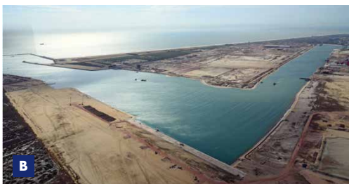
A Location and influence area of Port of Açu (source: Prumo) B Areal view of the areas 1 and 2 and access navigation channel
