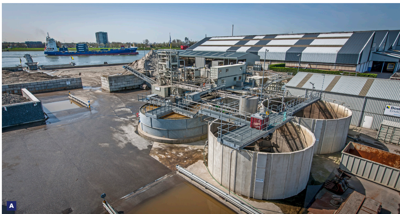
A Soil treatment installation in Schiedam
