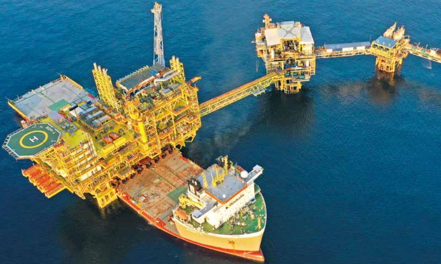
The semi-submersible heavy transport vessel Forte completed an incredibly precise float-over installation offshore the Malaysian part of Borneo in August 2020. The accurate positioning of the 11,238-ton Bokor CPP-A topside was the climax of a major project involving colleagues from various disciplines at Boskalis.
