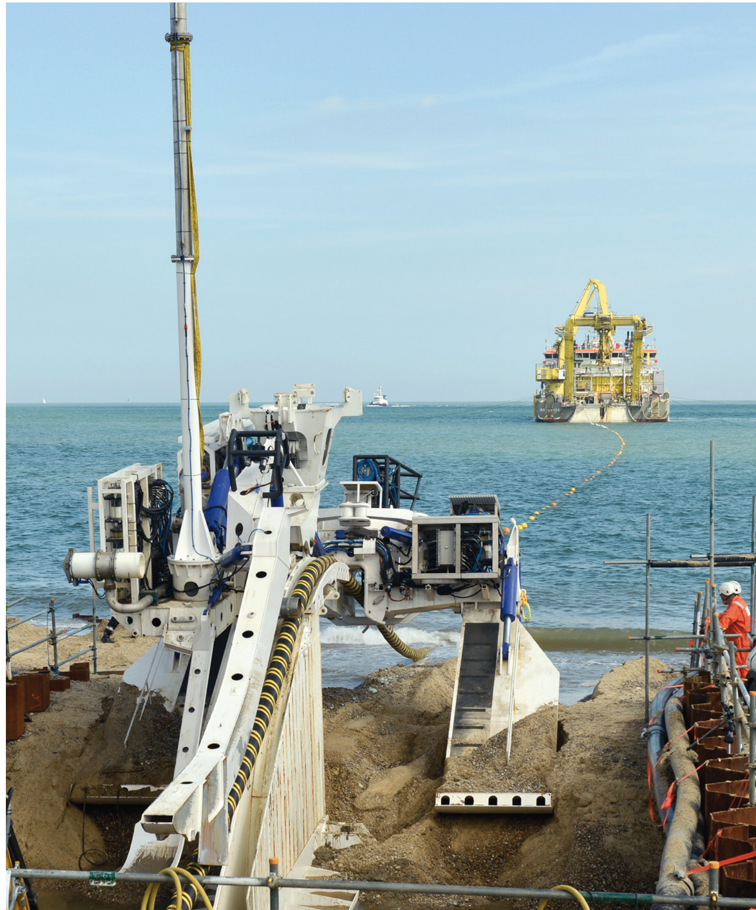
Shore landing of export cable by cable laying vessel Ndurance and HD3 plough
