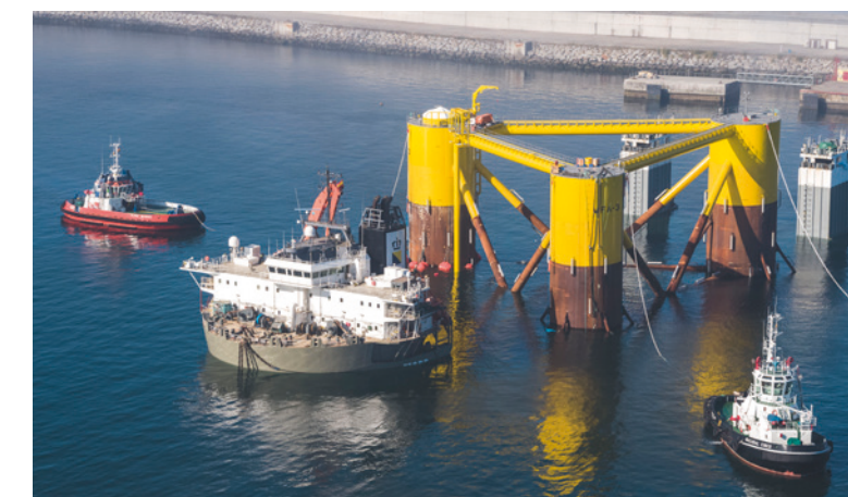
Floating foundation being submerged by semi-submersible barge Fjord
