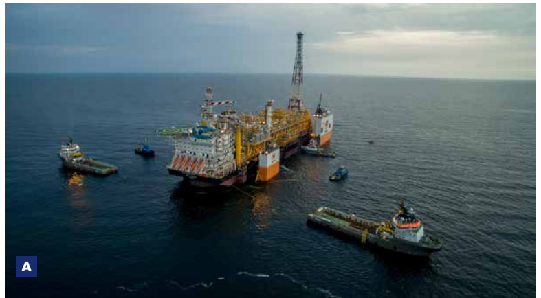
A Float-off operation at Port Gentil, Gabon. View from stern.
