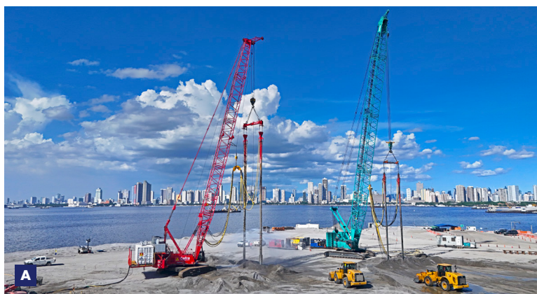
A Vibro Compaction works in tandem rig configuration. B TSHD Prins der Nederlanden discharging sand at the Project Site.
