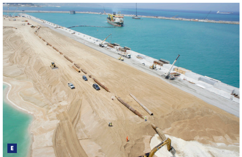
D Overview of the Tanger Med 2 port construction
