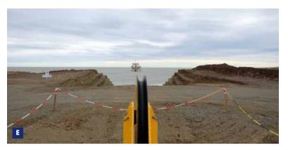
tolerances, in less than one day under difficult conditions. After confirmation and approval of the pull wire's position in the trench, the 1200 m pull commenced was completed successfully despite severe weather conditions.
