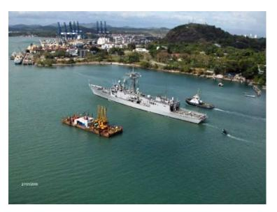
This operation went very smoothly and at no time did we interfere with canal traffic. On this project it was of vital importance to be able to deploy, blast and re-deploy the drill barge very quickly.
