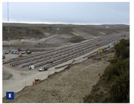
the northern landfall an 800 t linear winch system was installed to accommodate an 800 m pull-in of the pipeline from Allseas' pipe-laying vessel Solitaire. The winch was anchored by three Boskalis developed anchor moles with a 300 t holding capacity each. After the pull-in the Solitaire laid about 30 km pipeline towards Cabo Espíritu Santo, where the pipeline was laid down at the tie-in point.
