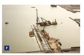
uniform underwater erosion protection features in front of the quays. They were made as underwater concrete works.
