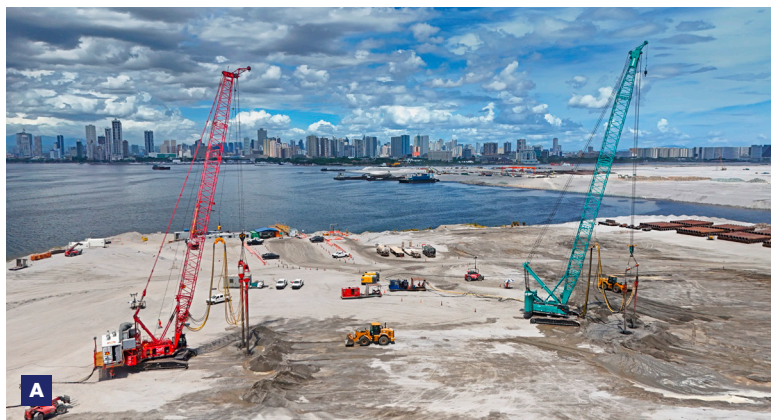
A Vibro Compaction works in tandem rig configuration.
