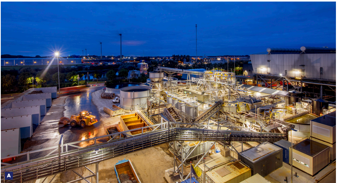
A The incinerator bottom ash (IBA) washing plant, in Alkmaar
