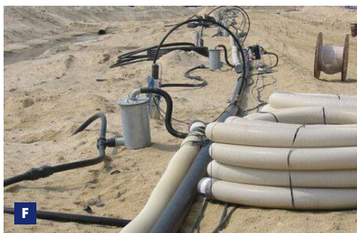
E Installation of the vertical barrier F Dewatering system G Installation of the vertical drains H EGTL site after completed ECP works
