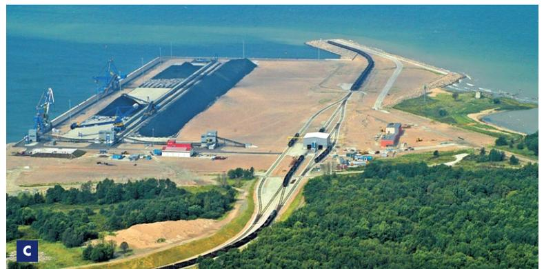
The two trailers completed the initial phase of dredging works by early February 2004. At that point, they had finished the reclamation and about 65 per cent of the dredging in the access channel. These operations were completed only six days before the Gulf of Finland became ice-bound. It was then that the Muuga construction effort focused on piling and associated tasks across the reclaimed area.
