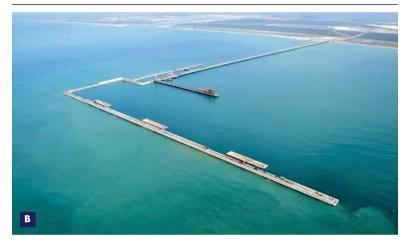
In this project, among others, the equipment used was: TSHD Oranje, TSHD Prins der Nederlanden; TSHD Willem van Oranje and Terra Plana multifunctional vessel. Reaching a total of 32,531,825 m³ dredged material. The dredged material was deposit in an oceanic drop zone, specified by the customer and as indicated in the environmental license, at a distance of 14 nautical miles.
