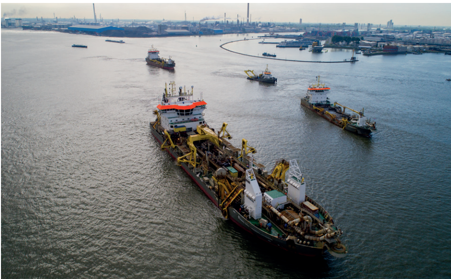
| Trailing suction hopper dredgers Prins der Nederlanden, Strandway and Causeway on the Nieuwe Waterweg & Botlek Deepening project
