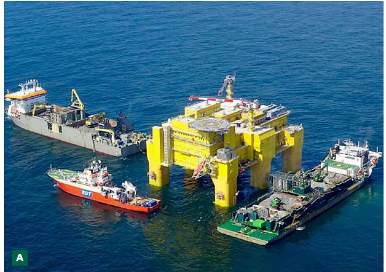
A Dolwin 2 project offshore positioning services B Boskalis Hydrographic survey vessel
