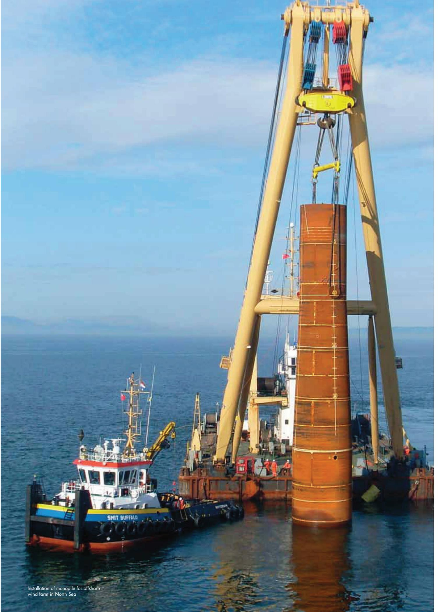
Installation of monopile for offshore wind farm in North Sea
