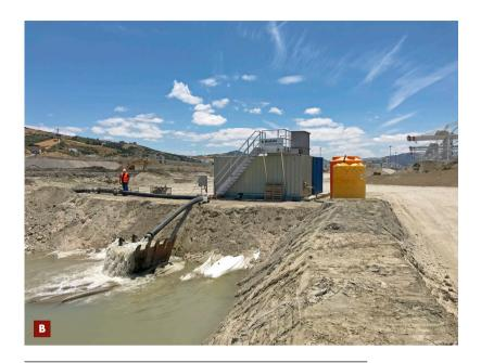
The dosing unit is equipped with a PLC system that enables remote control. For polymer bag change and Maintenance, staff is required on site. For this staff, no knowledge about the sedimentation process is required.
