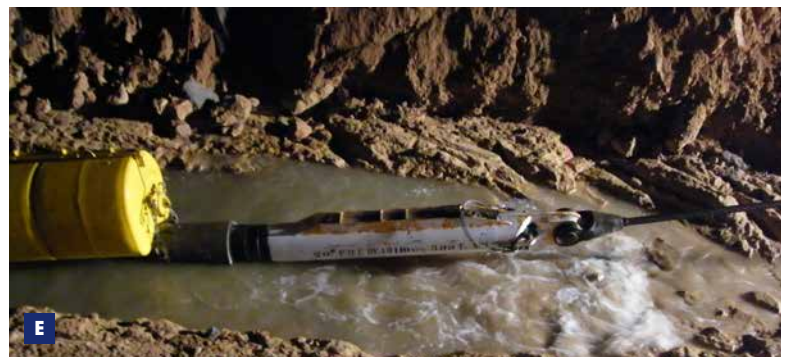
D TSHD Barent Zanen backfilling at Denia E Pipe pull at Mallorca
