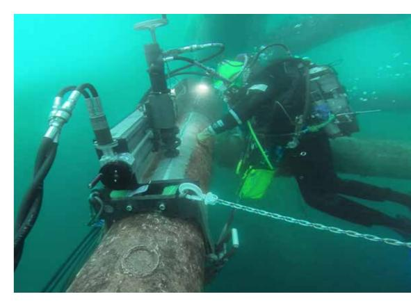
We pride ourselves on our ability to plan and execute high-quality IRM activity to subsea facilities. Whether it's targeted repairs or replacement of components, our versatile fleet enables us to respond swiftly to emergent and critical requirements. We also excel in managing long-term frame agreements; our client-focused approach ensures we build strong, long-term relationships, resulting in trust in our services.
