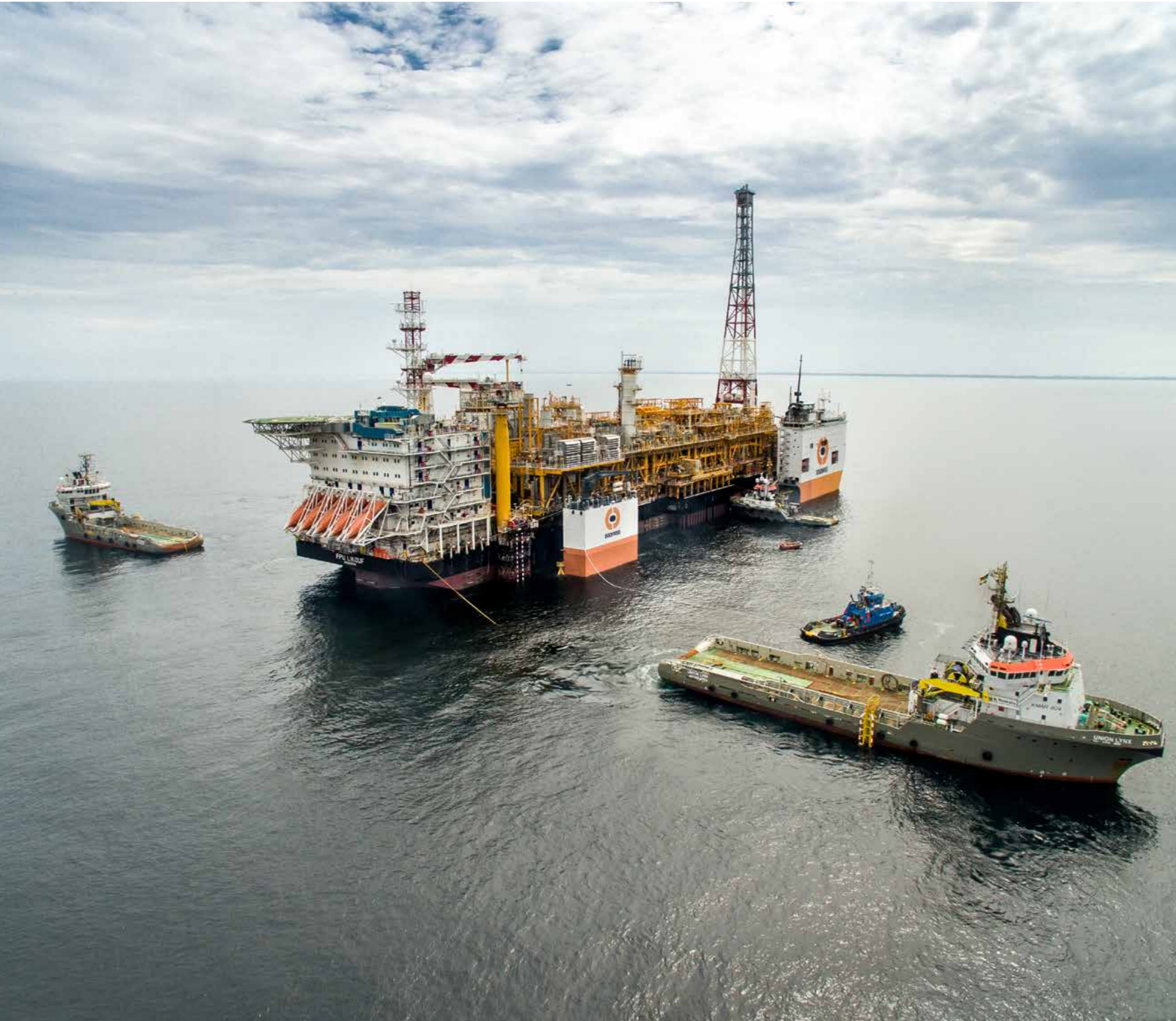
PORT GENTIL – GABON Float-off of the 80,500t Moho Nord FPU 'Likouf' from the Vanguard, supported by AHTs Union Lynx, Union Bear and Union Boxer, and Smit Lamnalco's Rima and Weaver.
