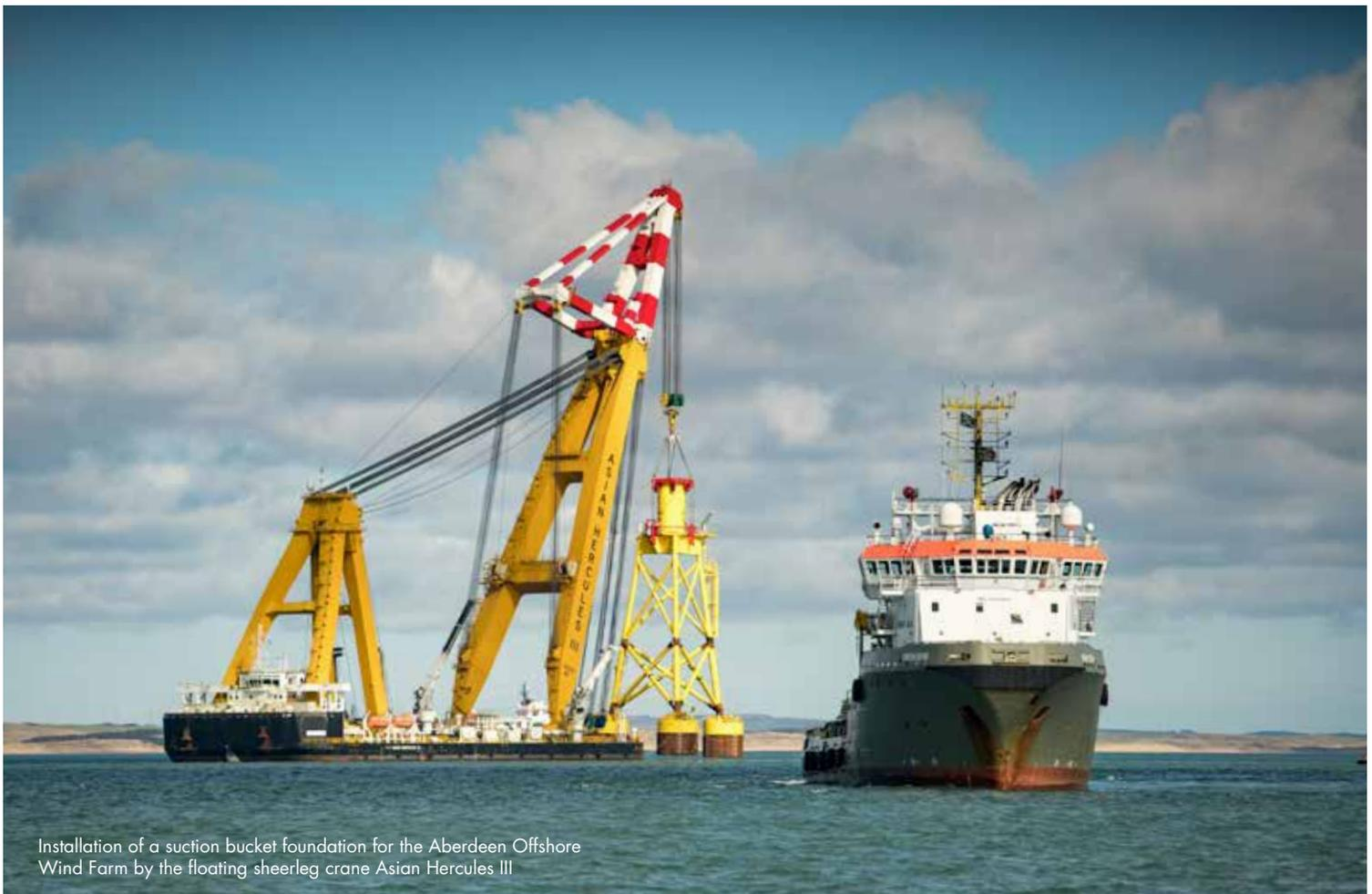
Installation of a suction bucket foundation for the Aberdeen Offshore Wind Farm by the floating sheerleg crane Asian Hercules III
