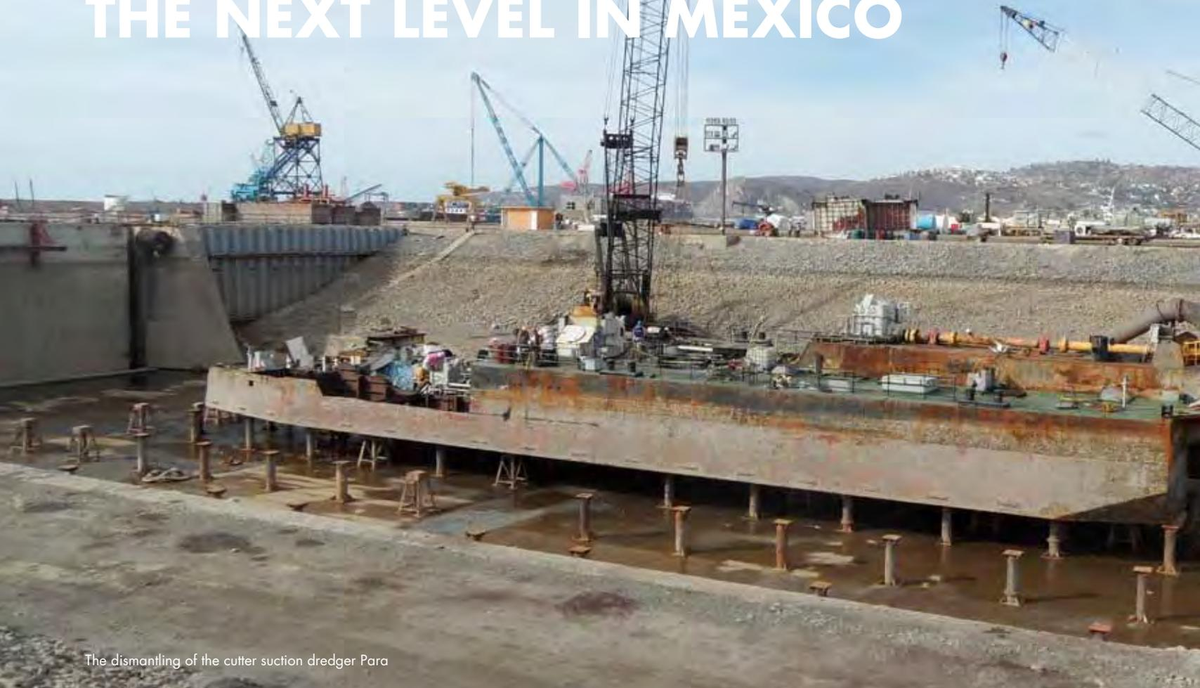
The dismantling of the cutter suction dredger Para
