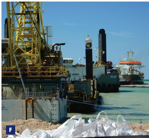
In front of the abutments a mooring facility was installed consisting of 7 dolphins connected by walkways. Each dolphin was constructed on steel pile frames, consisting of 1,750 tons of steel which have been grouted in drilled sockets in the seabed (1,240 m<sup>3</sup> of grout was used). 7 steel prefabricated dolphin jackets, consisting of 2,200 tons of steel and the connecting walkways were installed using a heavy lift vessel.
