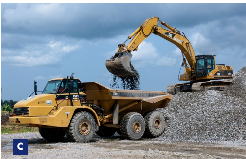
A Location map B Loading facility at Ogu Base C Laydown / Stockpile Area Ogu Base
