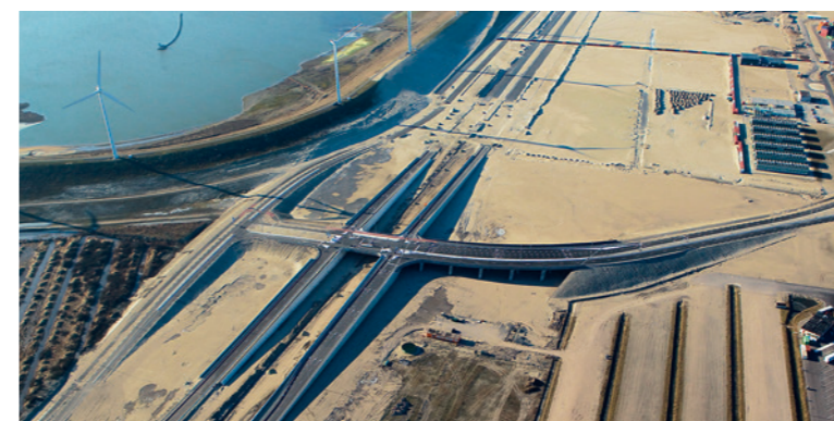
left ROTTERDAM, THE NETHERLANDS Design and construction of a retaining quay wall on the Maasvlakte 2 project. The project encompasses the construction of two innovative deep-sea quay walls, each 1.2m thick and 40m deep, and two quay walls for inland shipping vessels.
