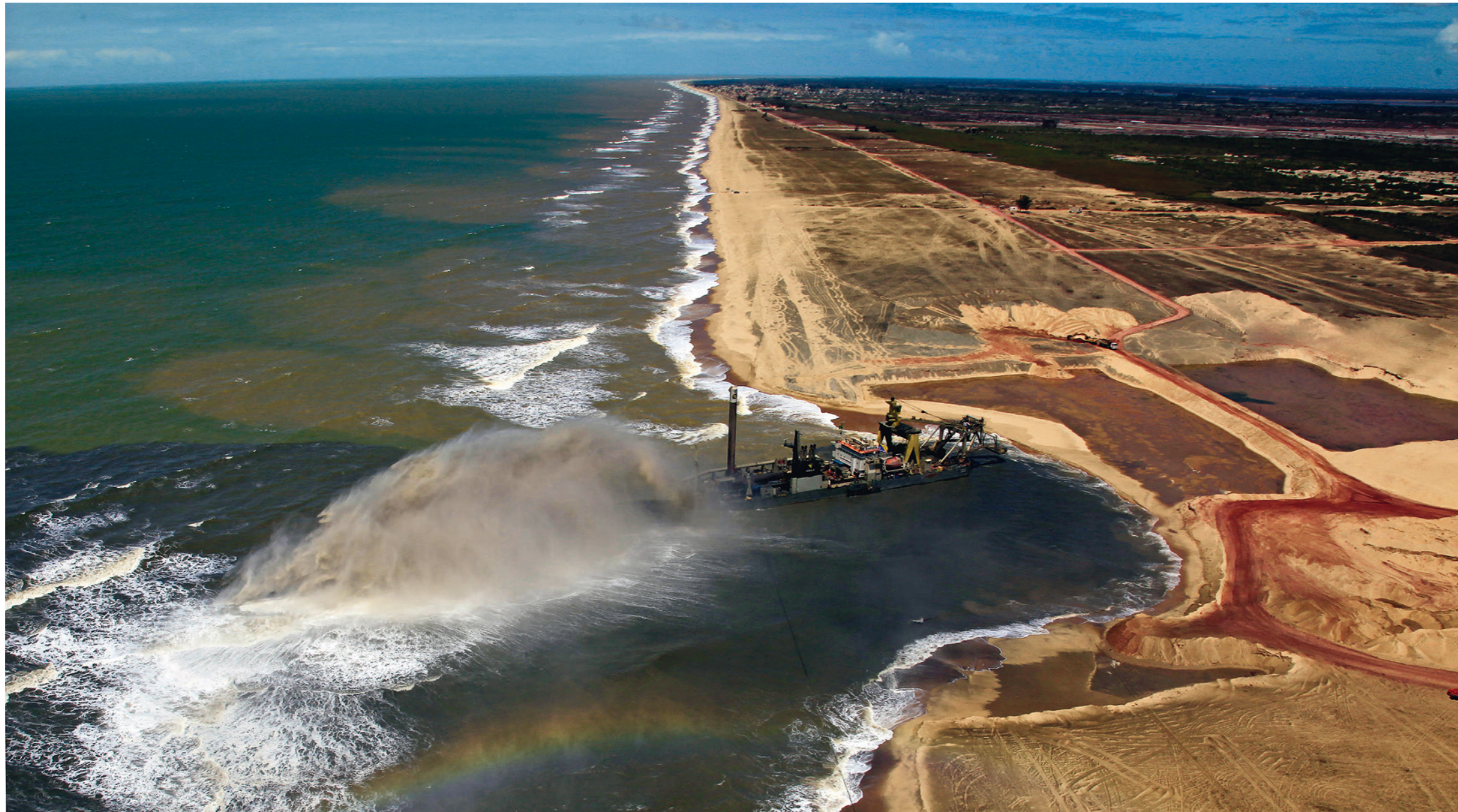
AÇU, BRAZIL The break-in operation through the surfzone at the beach for the access channel to the TX2 terminal at Superporto do Açú. The scope of the project includes the dredging of an access and inner channel, turning and port basin as well as land reclamation work. Boskalis will also construct the revetments at the entrance of the port.
