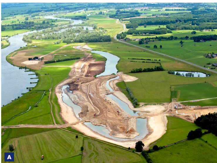
A excavation Munnikenhank
