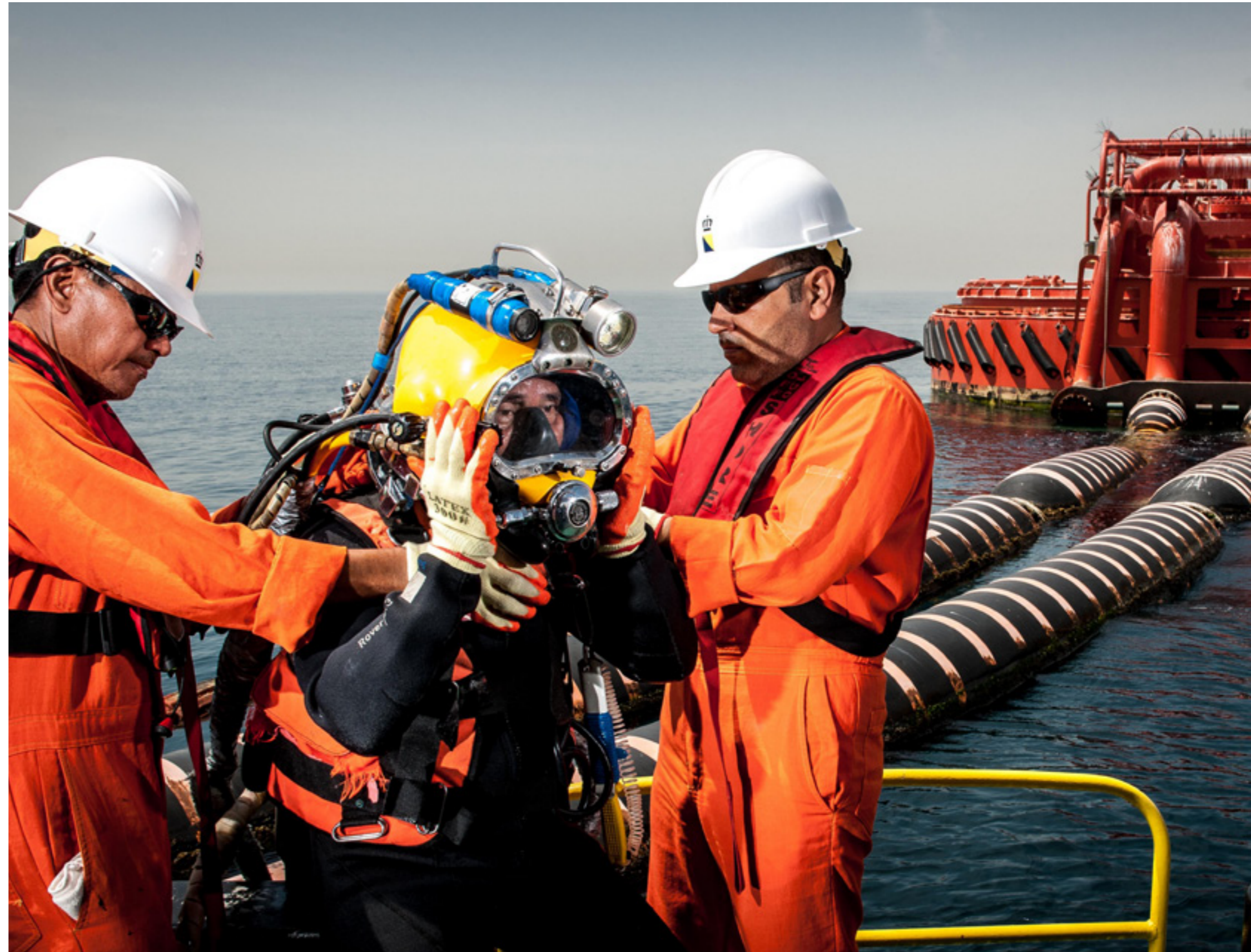
QATAR Air diver pre-dive check for maintenance work at a single point mooring buoy.
