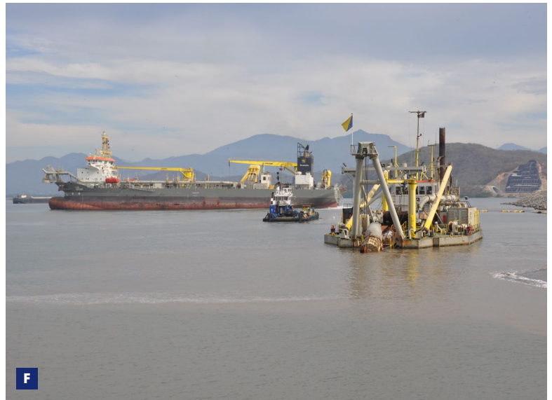
F Dredging of access channel by TSHD Gateway and CSD Para
