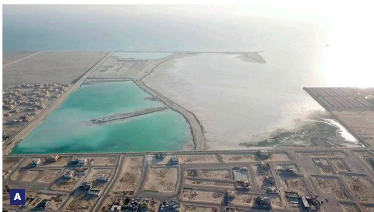
A Reclamation progress. B Dredging operations CSD Taurus II.
