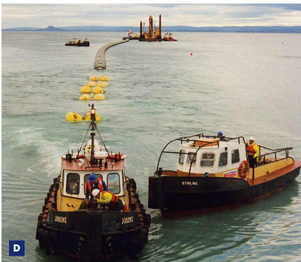
C Backhoe dredging ahead of landfall trench D Pipe Stringing in progress
