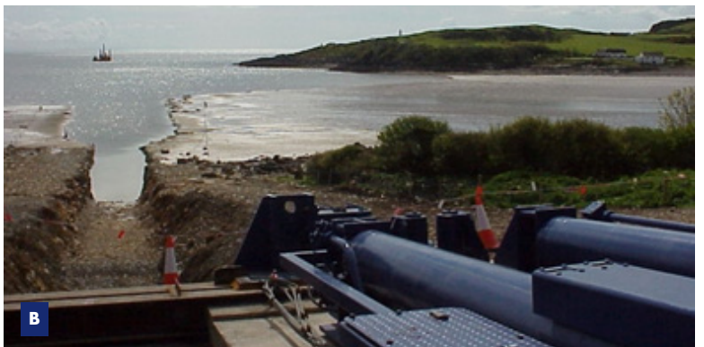
A Backhoe dredger preparing trenching for pipeline B Landfall showing pulling system
