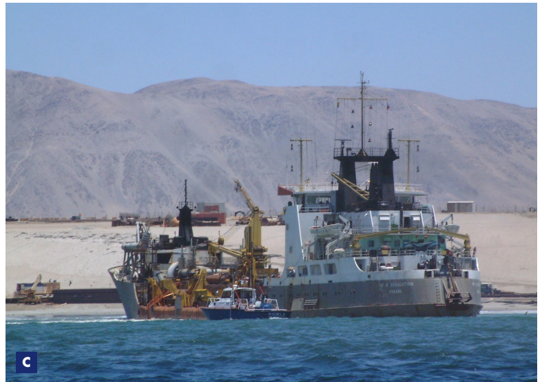
C Resolution dredging in the deeper areas
